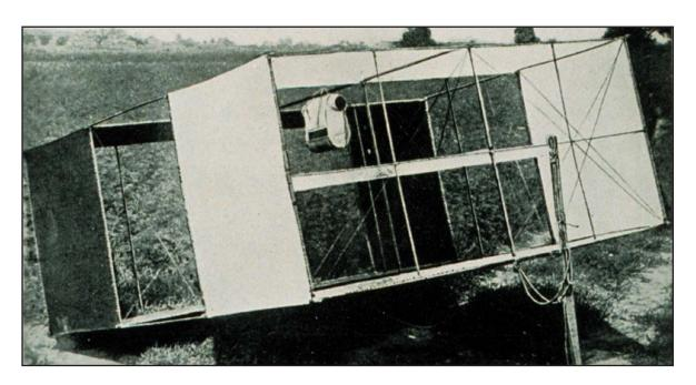
Weather kites carried scientific **instruments** into the sky. They recorded wind speed and temperature high in the clouds.
